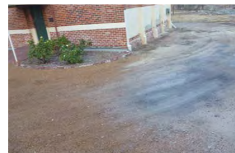
Vehicle activity blurring of the extents of the loose gravel parking area.
