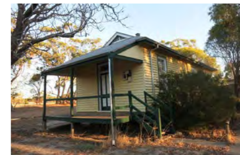
Former Police Station.
