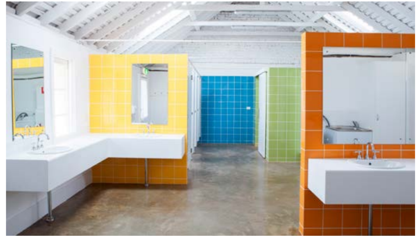
Bathroom Renovation at 'Our Barn', York
