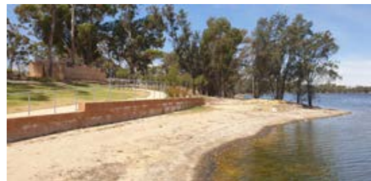
The natural environment of the Lake Foreshore is both fragile and harsh, and care must be taken to mitigate risks both to the Lake area, and to buildings located within it's environs.
