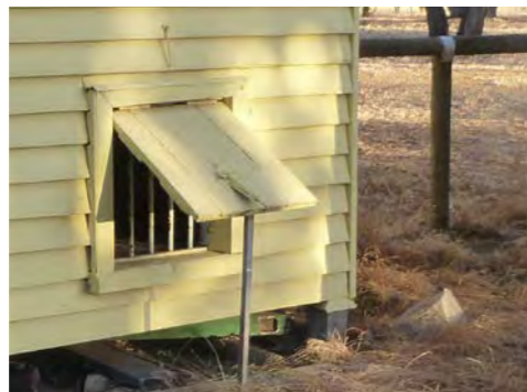
Iron bars can be seen across some windows and hint at the building's past.
