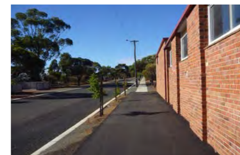
A clear but long, straight and ultimately uninviting path.
