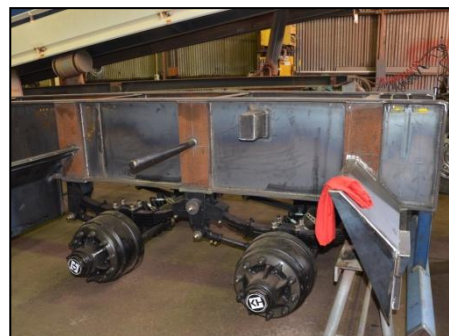
Photos of new trailer under construction
