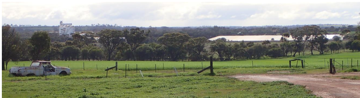
CBH Wickepin Receiving Site August 17 th 2022
