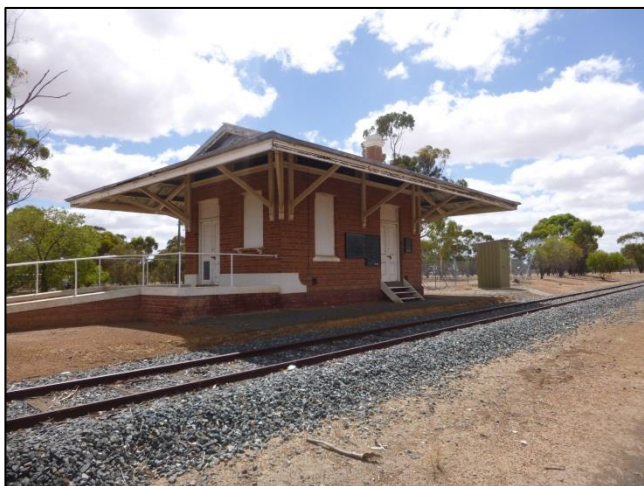
Wickepin Railway Station Office currently
