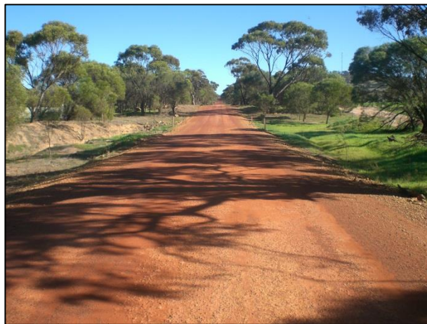
At slk 16.99 looking west through number four floodway highlighting the typical narrow road design
