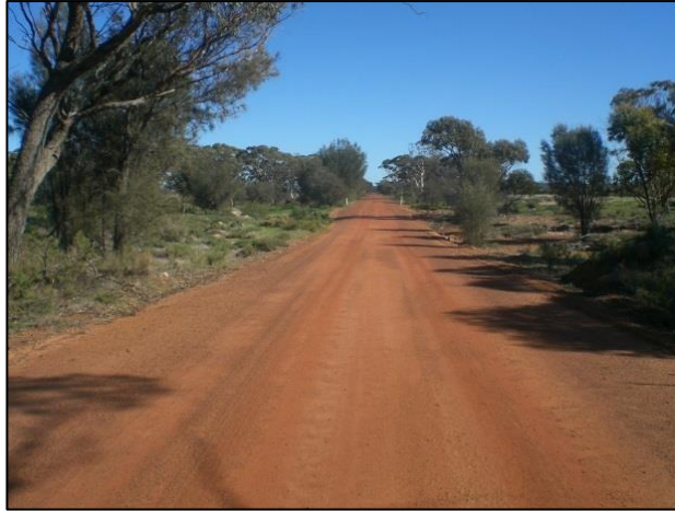
At slk 2.15 looking west through number one floodway highlighting the typical narrow road design
