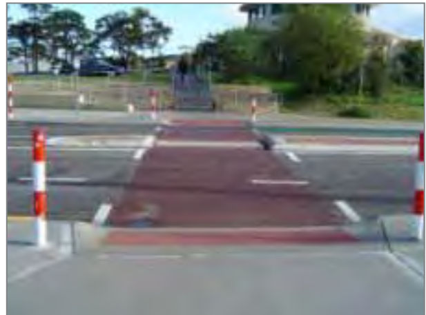
Stubbs Terrace, Shenton Park
