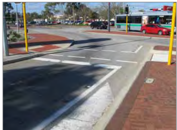
Albany Highway and Cecil Street
