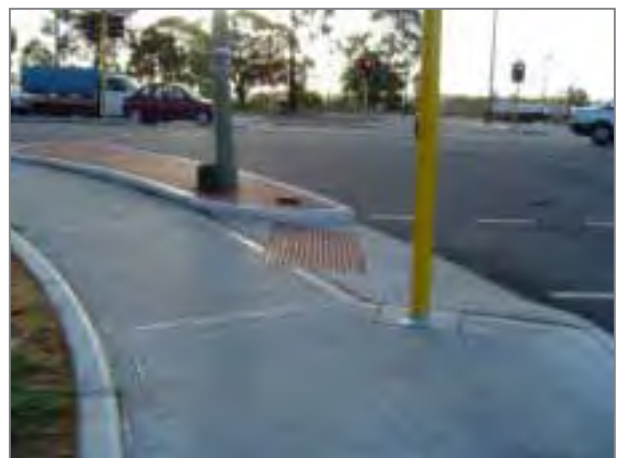
Correct Camber: Corner of Belmont Avenue and Great Eastern Highway, Belmont
