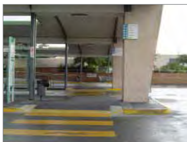
Booragoon Bus Station Note: The bottom photo shows that the sign should be mounted within the preferred range.
