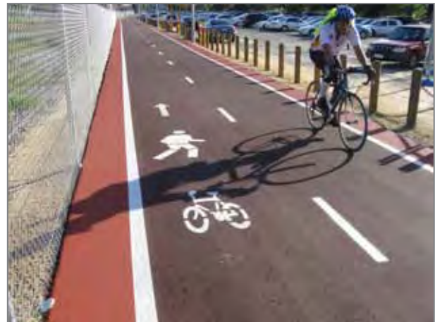
Shared path adjacent to Claremont Train Station
