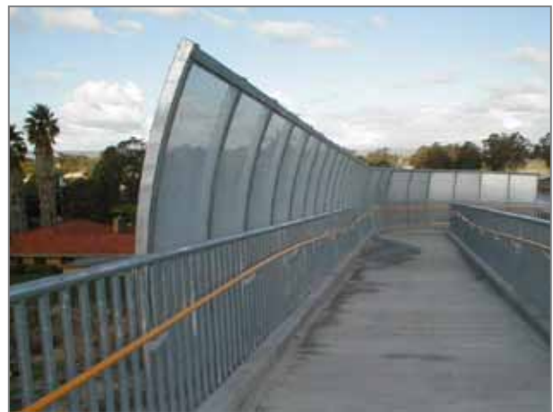
Barrier screen on Cameron Street Footbridge
