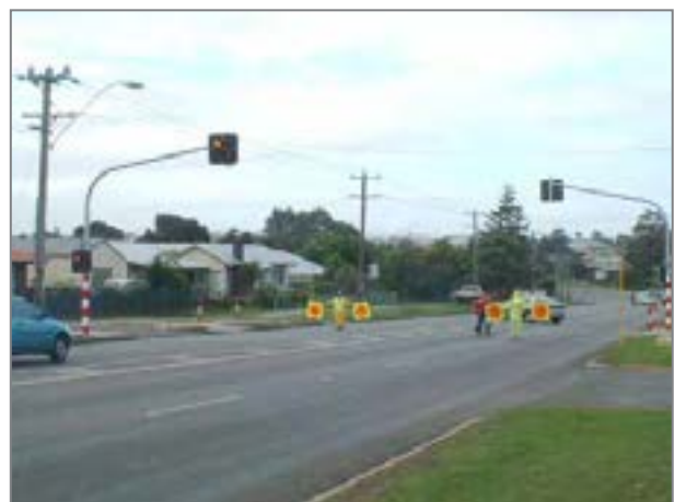
Albany Flashing Signal Crossing
