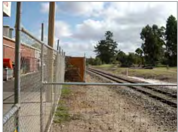
Visibility obscured by Storage Container
