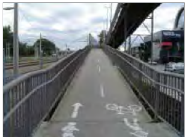
Roe Street, Northbridge, Pedestrian Overpass
