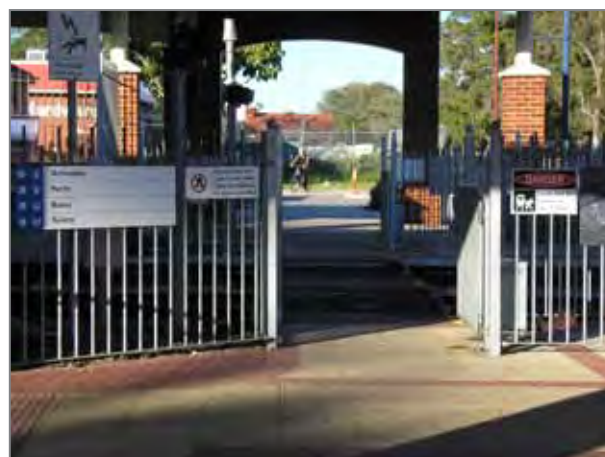
Gosnells Train Station Pedestrian Rail Crossing showing signage at correct height
