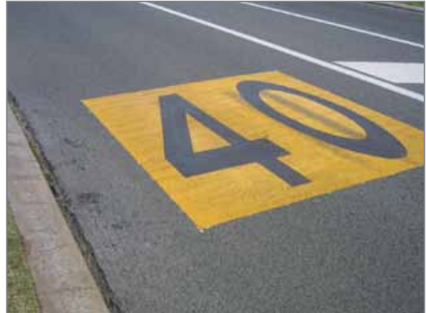
School Zone '40' Pavement Marking
