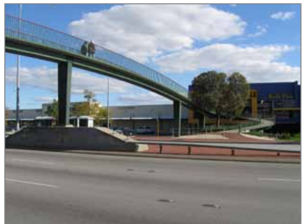
Pedestrian overpass at Carousel Shopping Centre, Cannington
