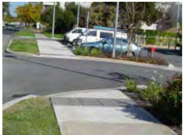
Hospital Avenue, Nedlands Example of a driveway serving large car park designed as an intersection (pedestrians give way to vehicles).
