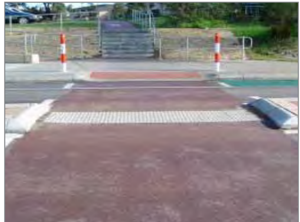
Stubbs Terrace, Shenton Park
