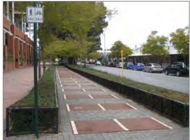
Separated Footpath and Cycle Path, Roberts Road, Subiaco
