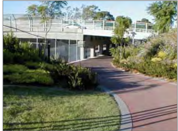
Underpass at Haydn Buntun Drive, Subiaco
