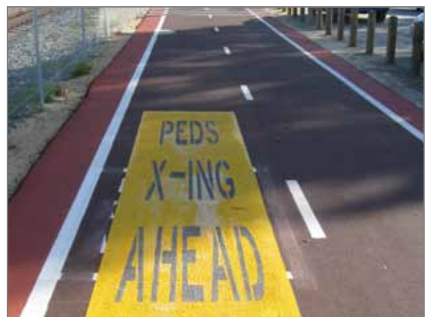
Claremont Train Station, treatment of shared path approach to pedestrian crossing
