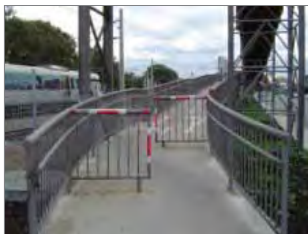
Pedestrian Overpass, Roe Street, Northbridge
