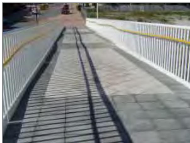
Pedestrian Overpass, Kwinana Freeway and Preston Street, Como
