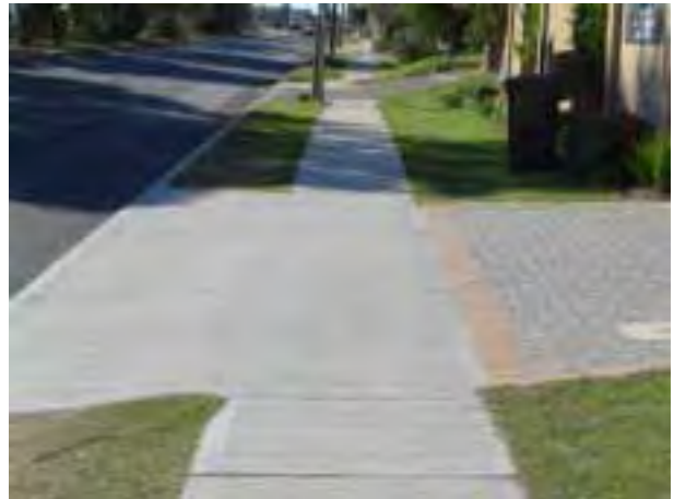
West Coast Highway, Scarborough Path continues across the driveway (vehicles give way to pedestrians)
