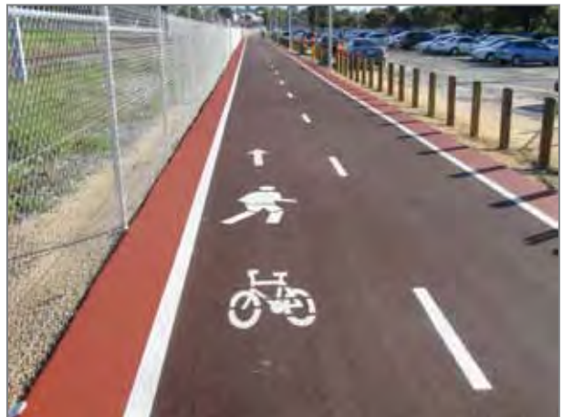
Shared path, Claremont Train Station
