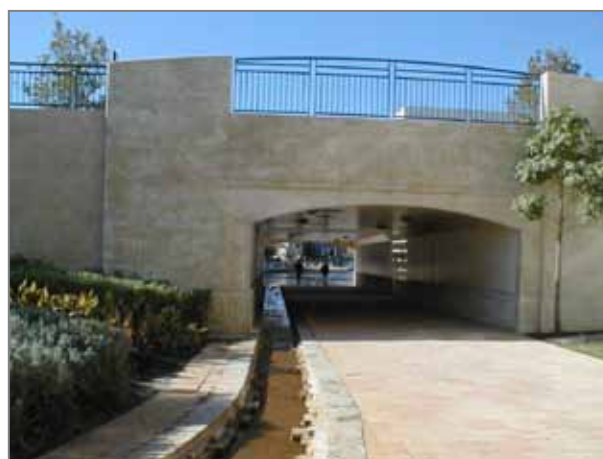
Underpass at Plain Street, East Perth
