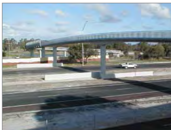
Footbridge at Roe Highway, Langford
