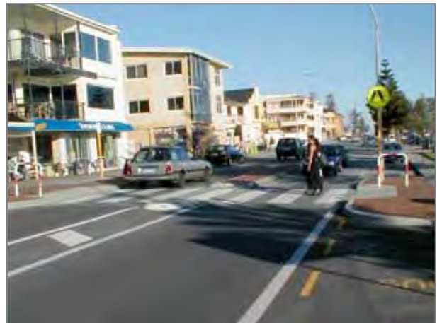
Marine Parade, Cottesloe Zebra Crossing, Kerb Extensions and Median Treatment
