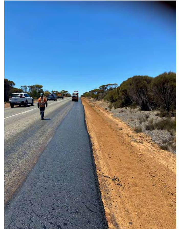
Asphalt widening Collie – Lake King
