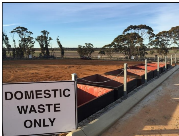
Tincurrin Waste Transfer Station
